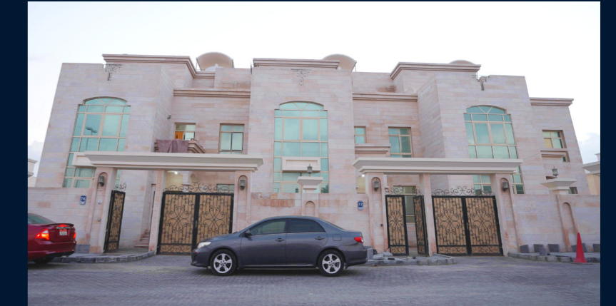
The company's business in Mohammed bin Zayed City also proceeded with the construction of three palaces (Al Mansouri 2-1) and a palace (Dr. Mazen).
