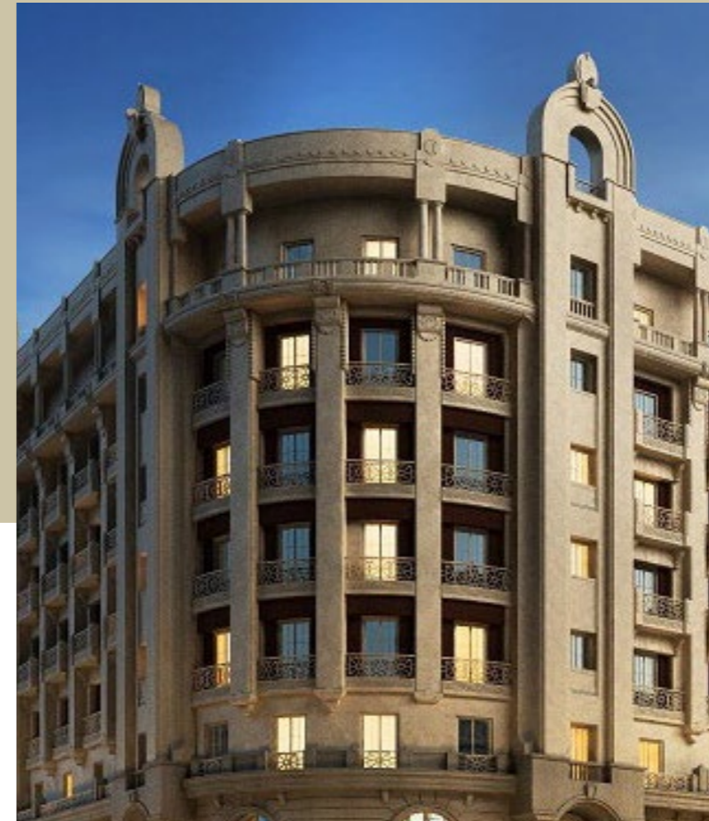
The New Capital Administrative Buildings
